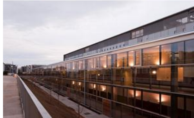
240: Daylight, views and ventilation, hospital Sant Joan Despi Barcelona
