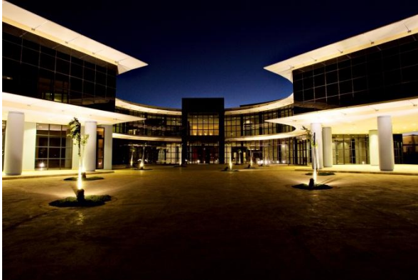
162: Main entrance, Vryburg Hospital, Northeast Province, SA
