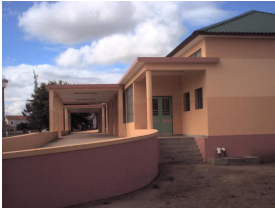
Figure 86: Single-story building, Chokwe rural hospital
