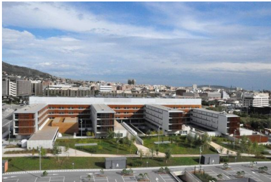
237: Overview of the hospital Sant Joan Despi Barcelona
