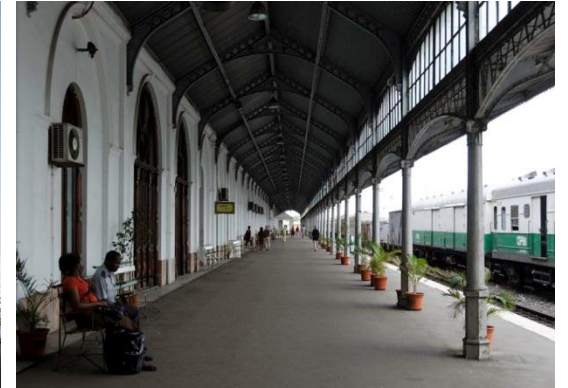
Figure 50: Maputo Railway Station – covered waiting station
