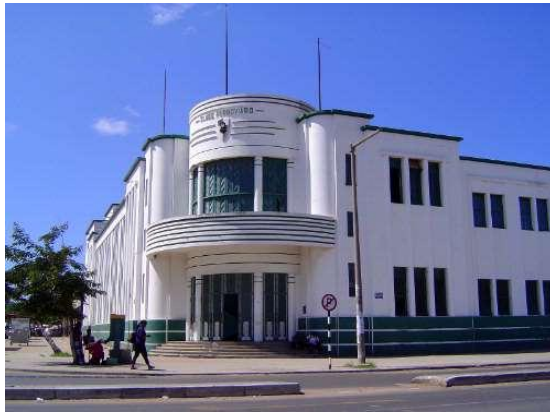
Figure 44: The railway club, Maputo down town
