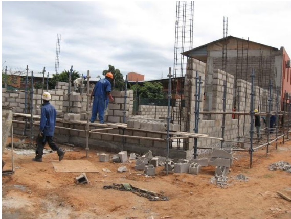
Figure 79: Conventional construction method, Mozambique
