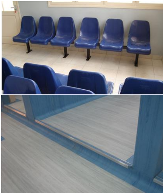
Figure 99: Tiles and vinyl floors: Clinical Lab, Beira Central Hosp.
