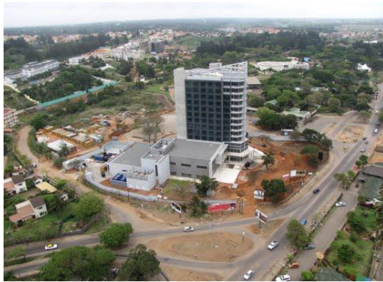
Figure 63: New hotel building under construction in Maputo
