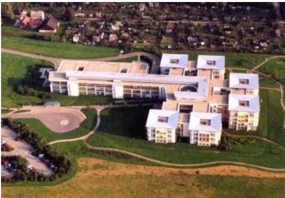
202: Community Hospital Chemnitzer Land, Hartmannsdorf, Germany
