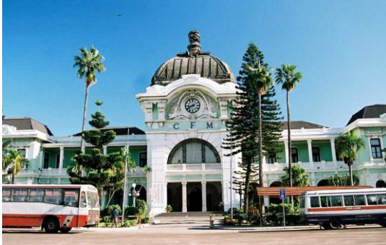
Figure 37: Maputo Railway Station designed by Gustav Eiffel, opened in 1910
