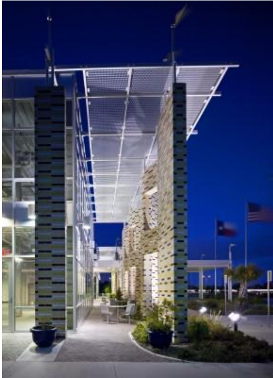
Figure 107: Driscoll Children's Hospital Pediatric Sub-Specialty Clinics, Texas
