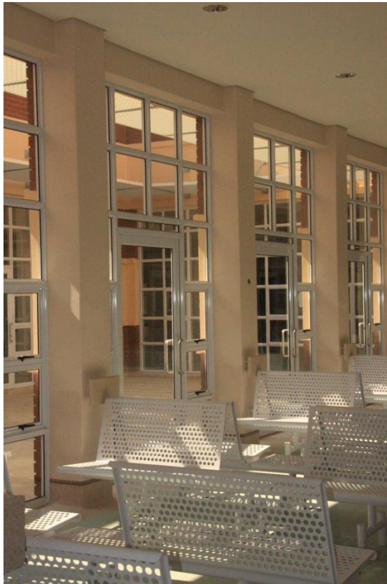
173: Windows & glazed doors along the waiting area – Passive Surveillance, Vryburg Hospital, SA
