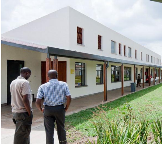
Figure 110: Building façade - windows to access daylight Butaro Hospital
