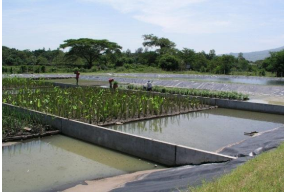
159: Constructed wetland, El Salvador
