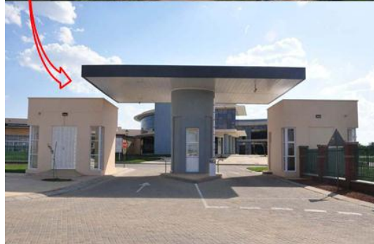
174: Controlled access - Fence & Main gate: Control access point, Vryburg Hospital, SA
