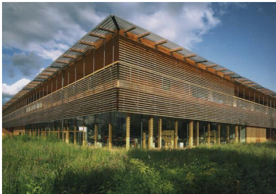
246: Building façades featured by wood material to provide thermal and sun control
