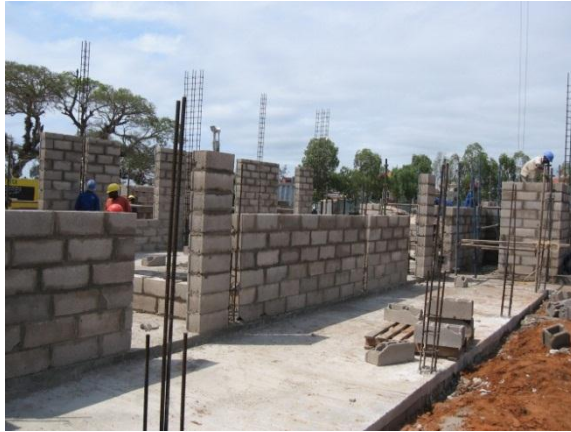
Figure 76: Walls construction: placement of hollowed cement blocks, Maputo Mozambique
