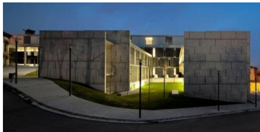
175: Defensive space - building façades, Hosp. Asilo of Granollers, Barcelona, Spain
