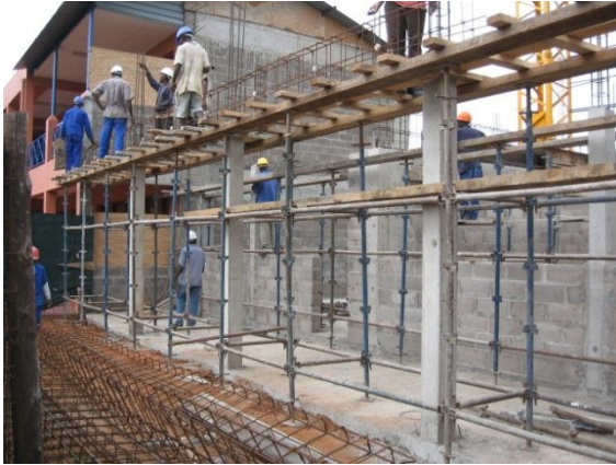
Figure 80: concrete elements reinforced and framework installation, site construction
