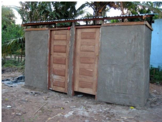
Figure 26: Improved latrine for the boys and girls in Chicumbane, Gaza province
